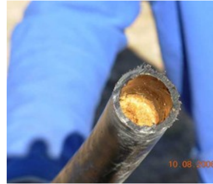
Pipeline: Before installing a Conditioner
