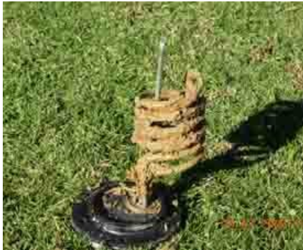
Hot Water Element: Before installing a Conditioner
