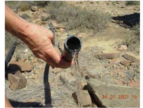
Pipeline: AFTER installing a Conditioner
